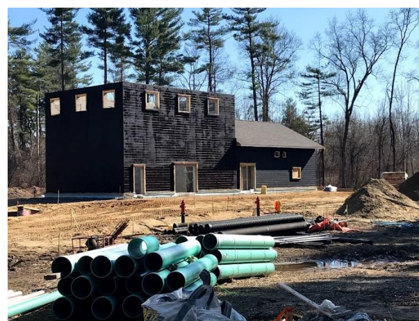
Figure 4 – Well 4 & 5 WTP Structure
