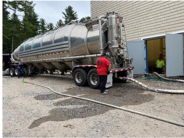
Figure 3-GAC Media Installation-Well 4/5 WTP
