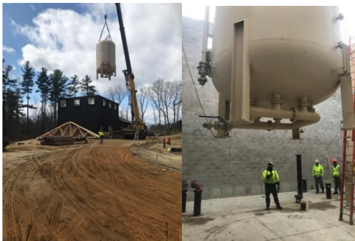
Figure 1-GAC Vessel Installation at Well 4/5 WTP
