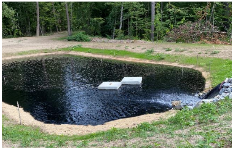
Figure 4-Initial Backwash of GAC at Startup-Well 4/5 WTP
