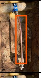
**Service Connection:** The portion of pipe that runs from the Water Main to the Curb Stop (refer to the orange rectangle in photo).
