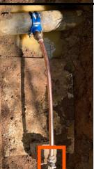
**Curb Stop:** Often referred to as the "outside shut-off or shut-off valve" the Curb Stop is the valve that connects the location's Water Service Line to the Service Connection. This valve allows the service location's water to be turned on and off as needed. The Curb Stop is located underground below frost level (approximately four to five feet) and is normally located at or near the service location's property line.
