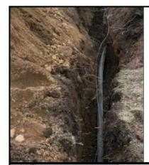
**Water Service Line:** The portion of pipe located underground that provides connection to water service. The Water Service Line is connected from Curb Stop into the premises.
